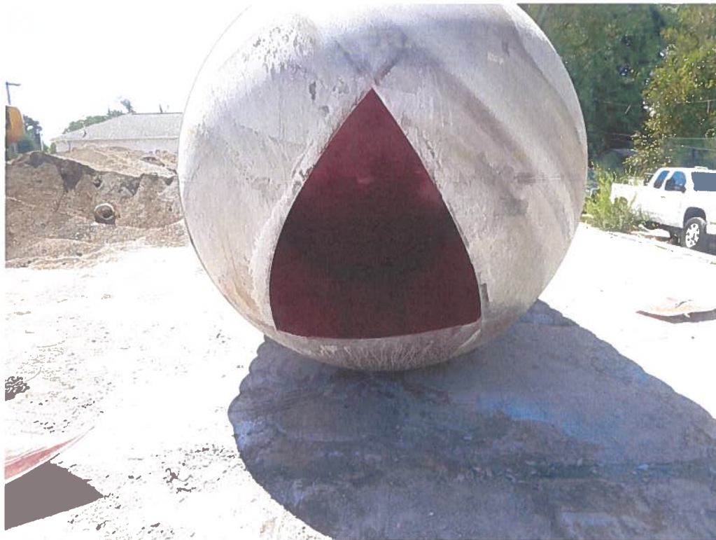
Date: 8/31/2022 Time: 11:52am Direction: S Photo by: Robert Mileur Exposure #: 014 Comments: Second UST cut open on north and south ends.
