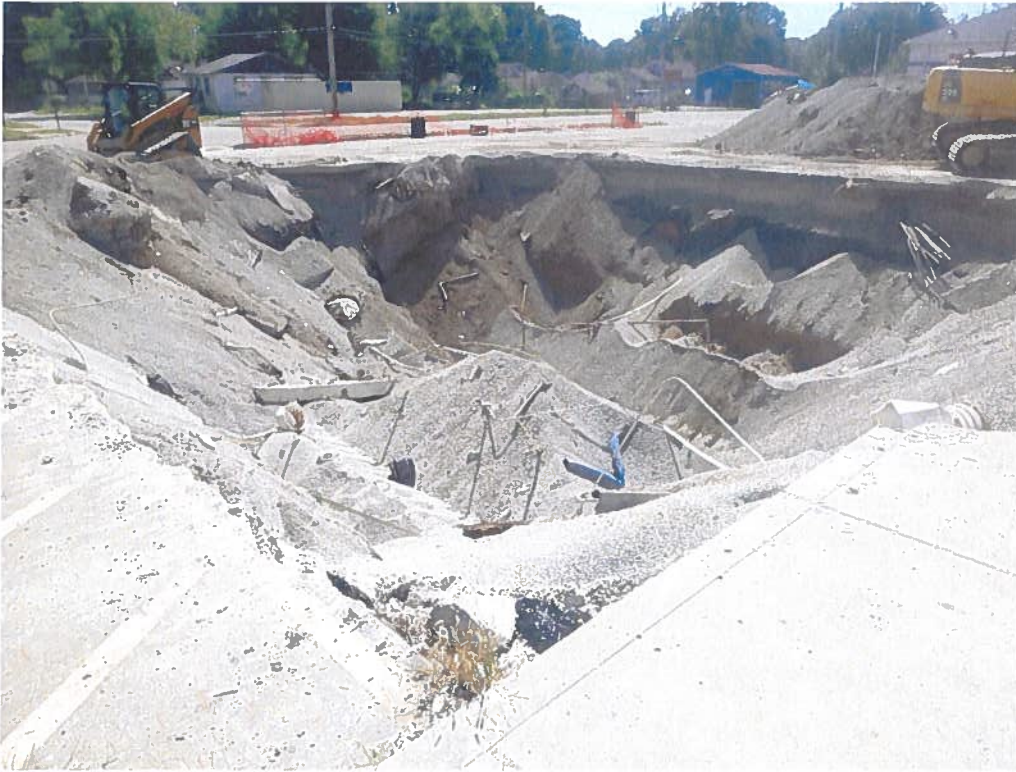
Date: 8/31/2022 Time: 11:18am Direction: NE Photo by: Robert Mileur Exposure #: 013 Comments: Tank field with both UST's removed
